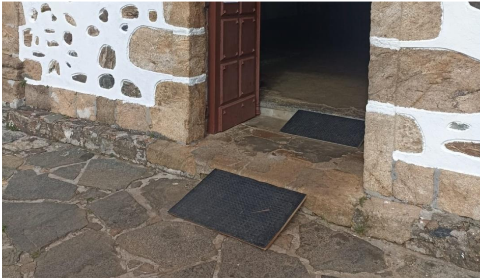
Figure 9. Access ramp to the sanctuary
